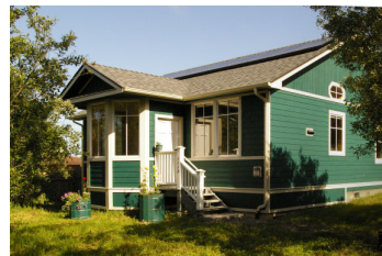
Fig. 2: South and east walls
